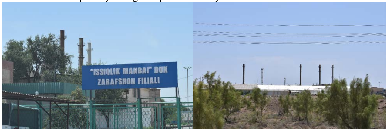
Figure 11. Photograph of the pipes of the city boiler house
